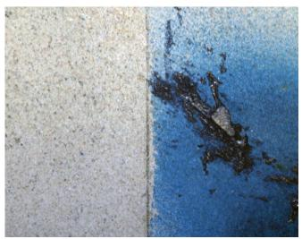
the wax and graffiti are removed together, sometimes with solvents or more commonly by melting the wax with steam or hot water. Once the anti-graffiti coatings have been removed, a new barrier coating can be applied again.
